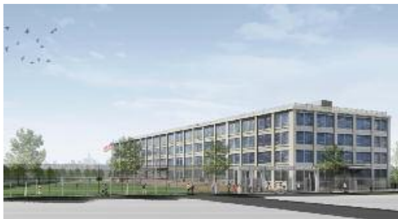
This newly renovated building in Elmhurst, Queens, is the home of BHSEC II for the 2008–09 academic year.
